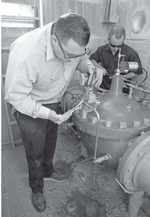
Dino Trujillo and Daniel West working on a pressure reducing valve.
